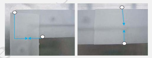
In the above images, the white circles indicate where 3M 4000UV should be applied in the corner and step situations. These two general categories can describe most common configurations. For configurations other than these, the general principle is to use 3M<sup>TM</sup> 4000UV in any place where water (shown as blue arrows) could seep past an improperly joined overlap.
